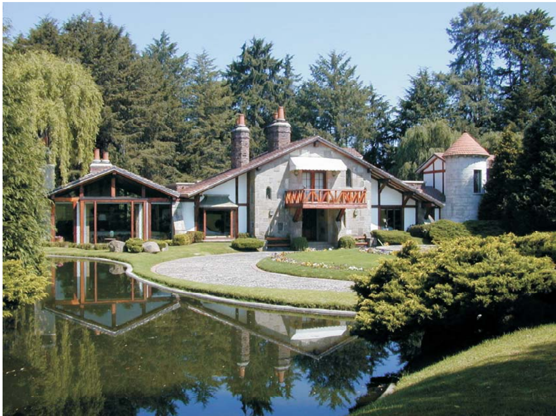
All interior and exterior glass was renovated and protected with the ClearShield System
