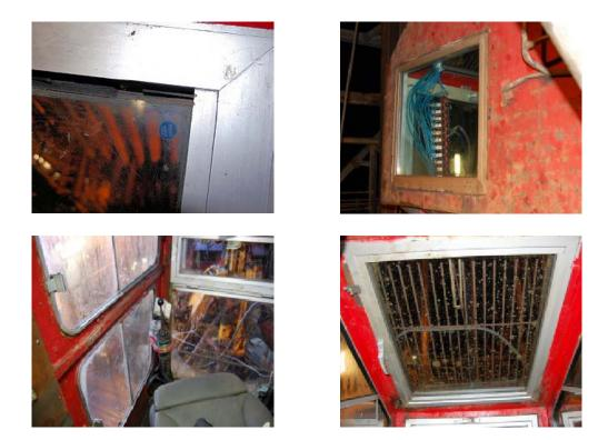
Some glass on the Deep Sea Bergen Oil Platform was treated with ClearShield 15 years ago to prevent glass corrosion (top row). Compare this with untreated driller cabin glass at the same installation (bottom row) – the difference is clear.
