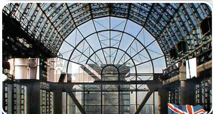
Lloyd's of London Building
