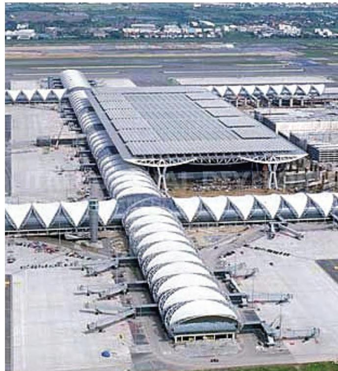
ClearShield helped to reduce costs and delays on the construction site of this new major airport by protecting the glass from cement, concrete and construction dust. Some 100,000m<sup>2</sup> of glass was treated.
